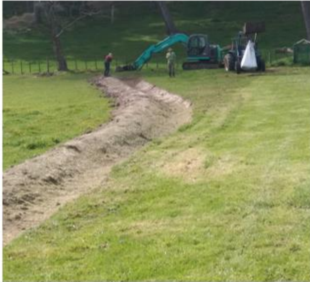
Constructing a swale
